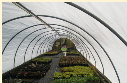
Figure 13. (top) Plants in a coastal plain ecoregion are pushed together beneath a structure covered with shade cloth. (bottom) An overwintering structure 22' wide by 96' long is covered with one layer of 4 mil white polyethylene. The ends are made of wood, and ventilation is created by opening the doors at either end of the house.
