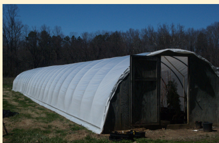
Figure 13. (top) Plants in a coastal plain ecoregion are pushed together beneath a structure covered with shade cloth. (bottom) An overwintering structure 22' wide by 96' long is covered with one layer of 4 mil white polyethylene. The ends are made of wood, and ventilation is created by opening the doors at either end of the house.
