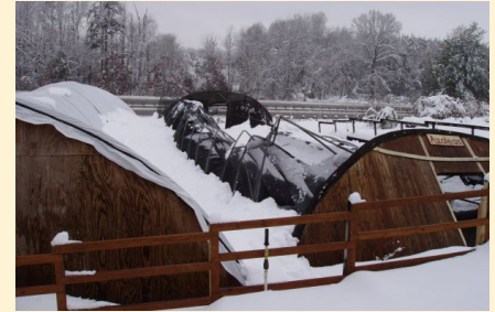
Figure 17. Winter protection houses collapsed by snow load. The greenhouse in the left-hand photograph and the greenhouse on the right side of the right-hand photograph were covered with shade cloth, which accumulates snow load more quickly than plastic. In this particular heavy snow accumulation, the house covered with plastic on the left side of the right-hand picture also collapsed, although not as severely. These collapses occurred within hours of snow beginning to fall.
